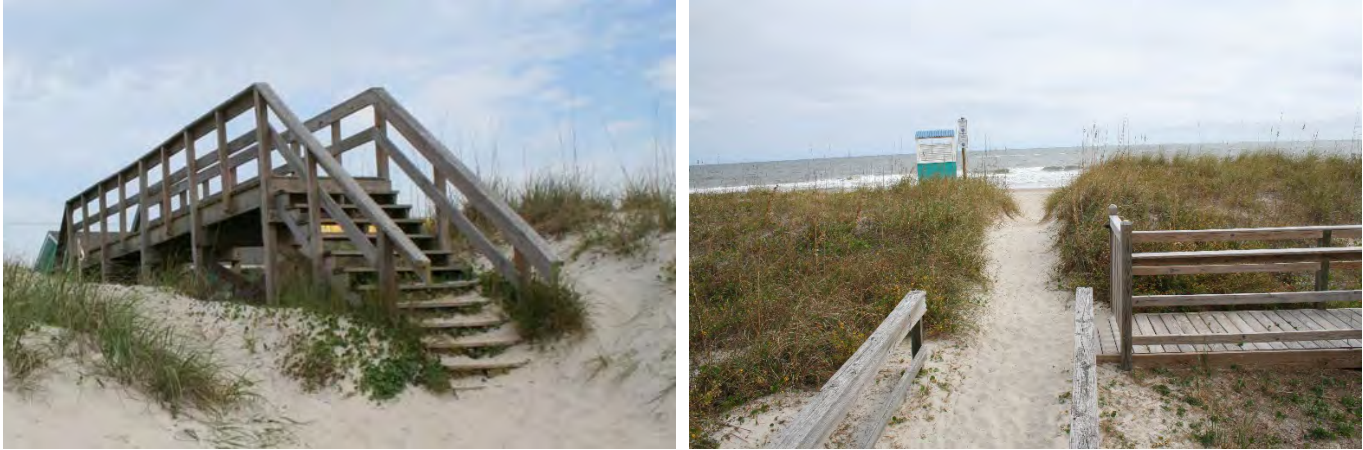
Figure 4. Typical Dune Access (Walkover Structure & Foot Path)
