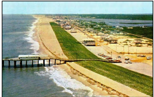
Figure 4 Carolina Beach post construction
