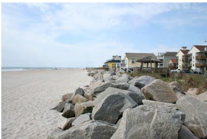
Figure 7. Northern Rock Revetment after the 2016 CSDR Maintenance Event
