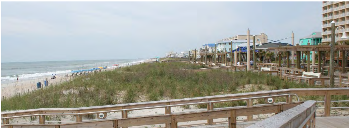
Figure 5. Carolina Beach Boardwalk & Primary Dune
