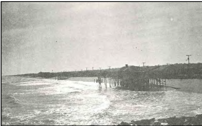
Figure 3 Carolina Beach pre-1964 construction
